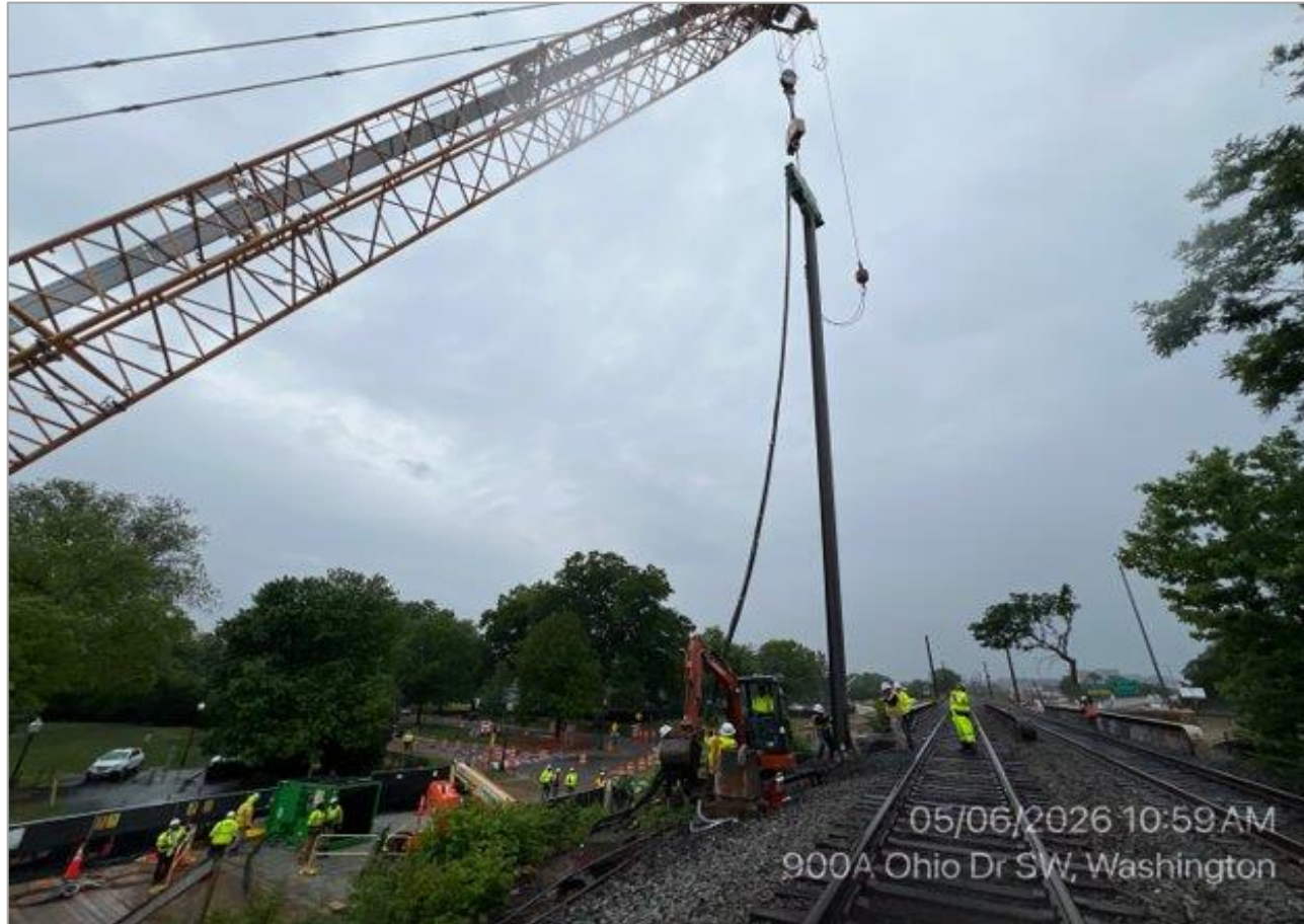
Ohio Dr. Bridge Support Of Excavation Pile
