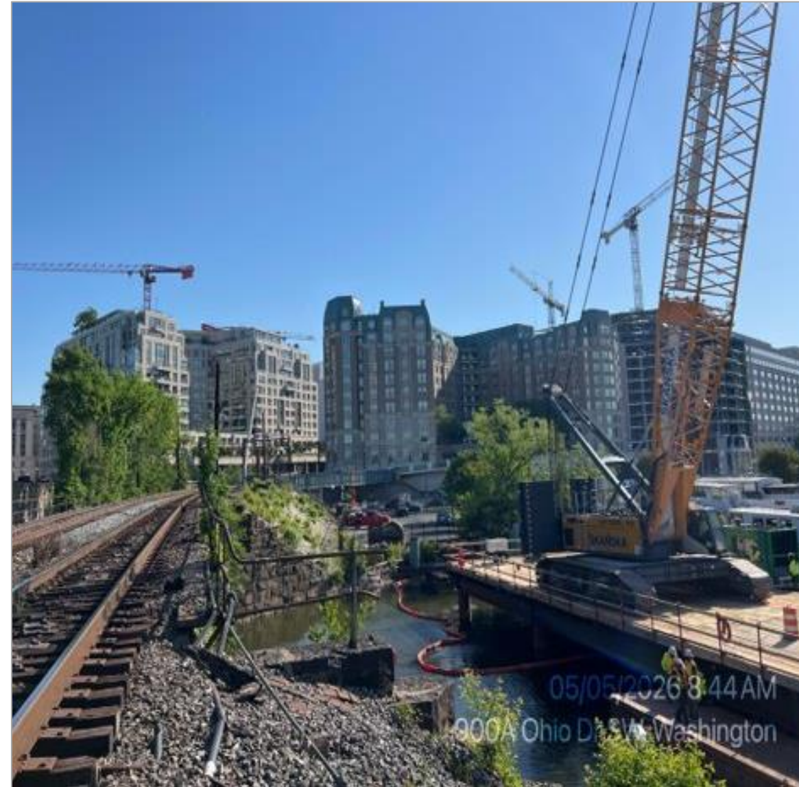
Trestle Construction at Washington Channel
