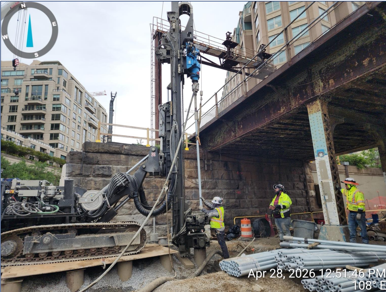
Micropile Installation at Maine Ave. Abut. B
