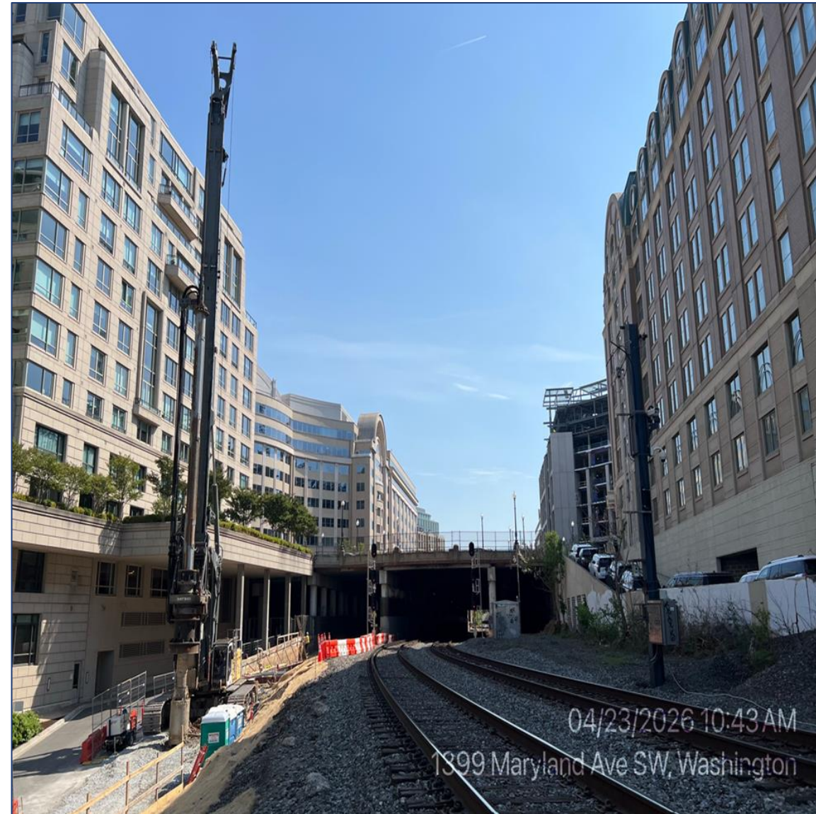
Drilled Shaft Installation at Retaining Wall L
